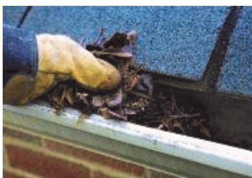
You can install "netting or sieve" on top of the gutters which will prevent any leaves from going into it (available at a hardware store)
